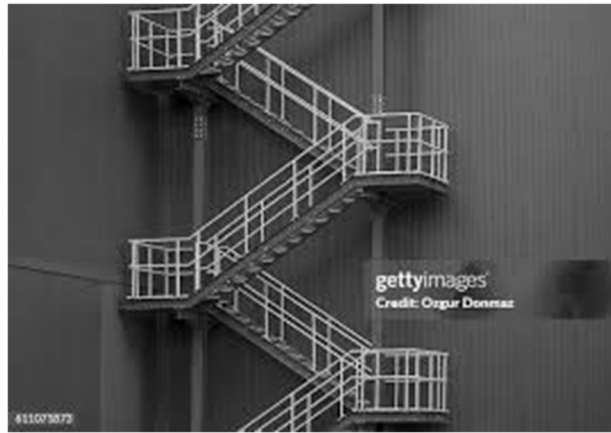
Factory stairs to multiple levels
